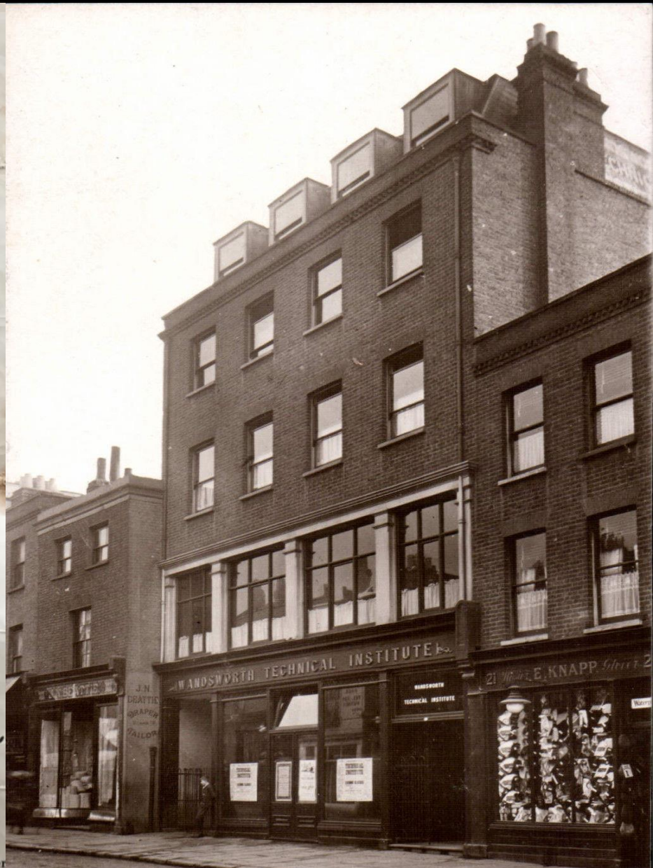
Wandsworth Technical Institute.
